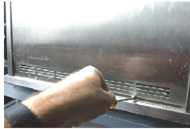
Figure 1: All units are disassembled in a similar fashion. Two screws, at the base of each side, secure the side panels.
